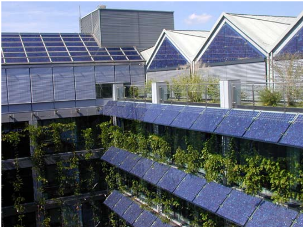
German Association of Savings banks Solar energy plant on one of BayernLB's buildings in Munich
