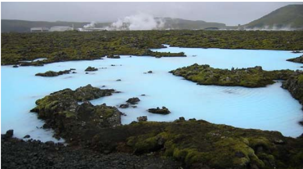
Hitaveita Suðurnesja Geothermal Powerplant in Iceland
